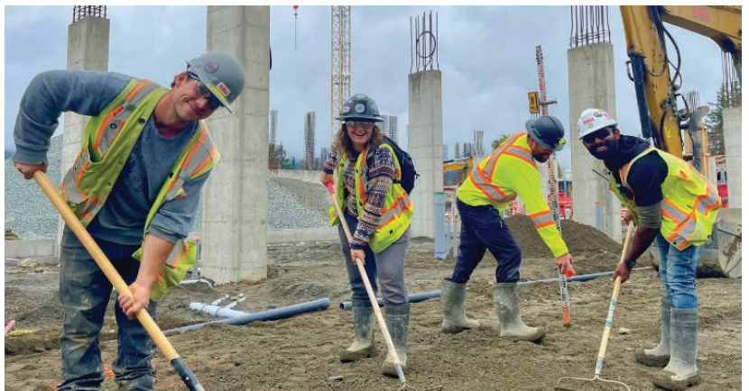
L-R: CDH Replacement site crew - Paolo, Jamie, Terre and Romi
