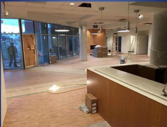
Millwork and Finishing work continues
